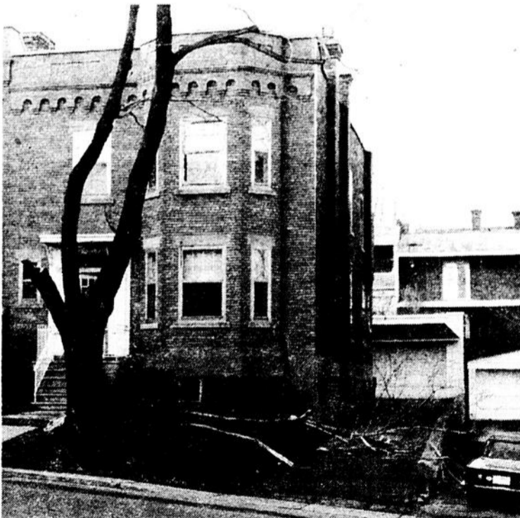
WINDY VICTORIA: High winds struck the area about supper hour Tuesday evening. Though no serious damage was reported in Westmount, there was a close encounter of the fallen tree kind at this home at 629 Victoria avenue. Just before this large and not-very-sound limb came crashing down across the driveway, an occupant of the house had driven his car out of the way on an errand. Only result was an upstairs window broken to be repaired and a lot of fir, poplar, wood to be cut up and stowed.
