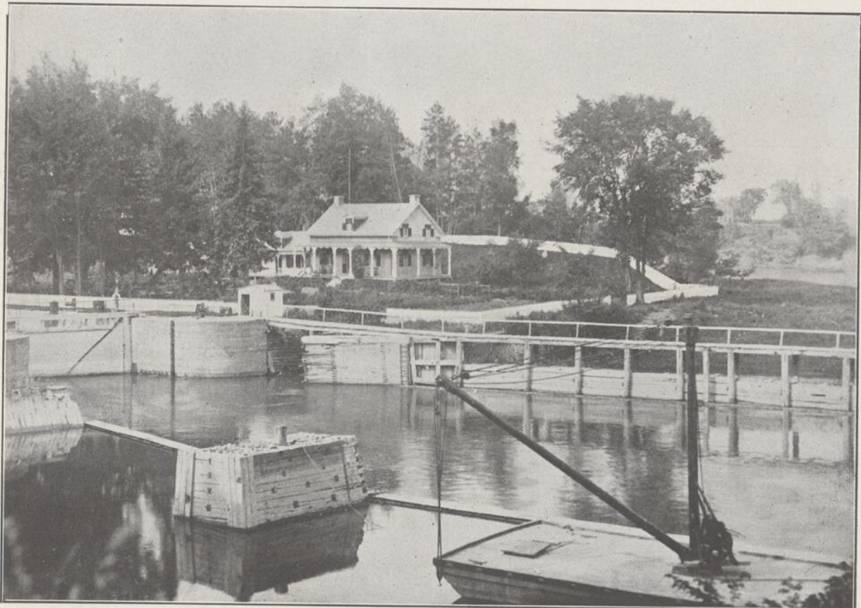
General view, looking south-west, at the St. Ours lock No. 66.
