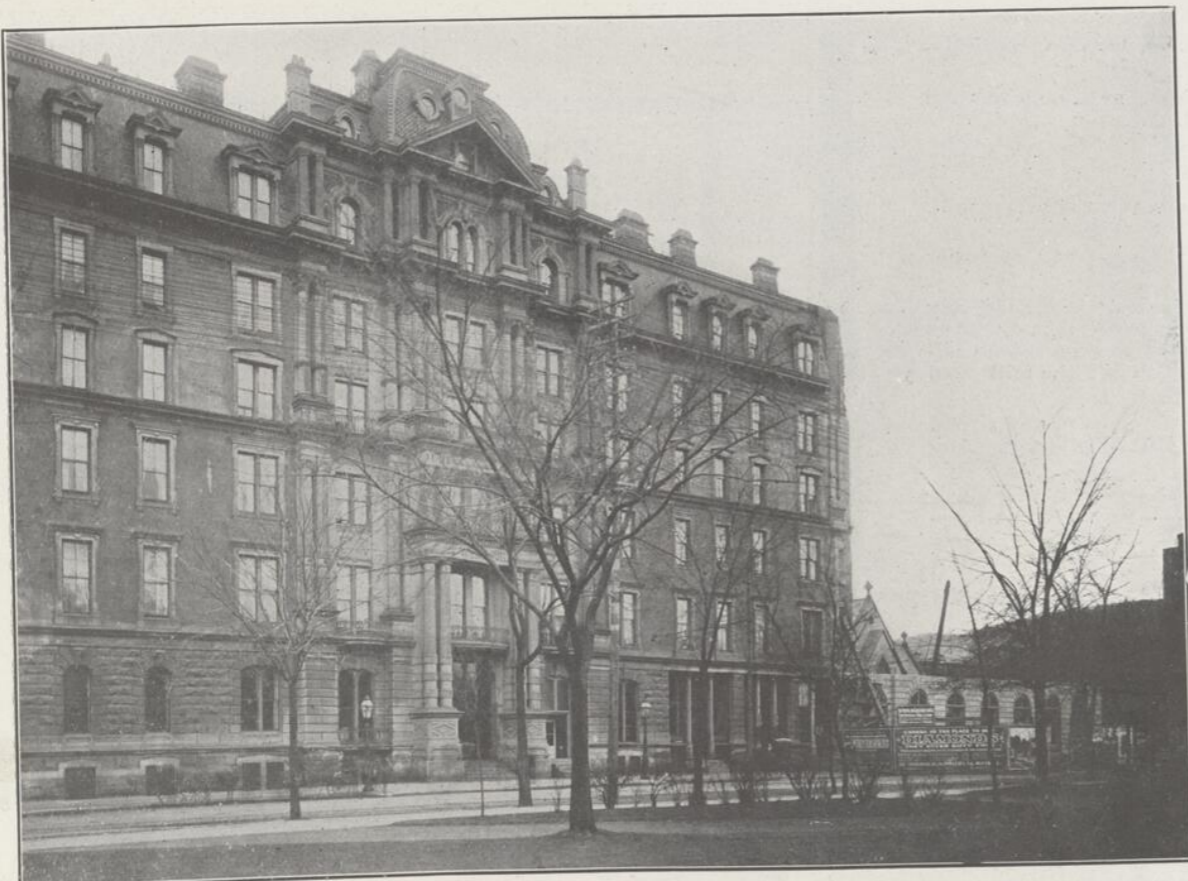
PROMINENT LANDMARKS ON DOMINION SQUARE, MONTREAL—The Windsor Hotel as it now is, showing the addition now in course of erection to the north of the main building.
