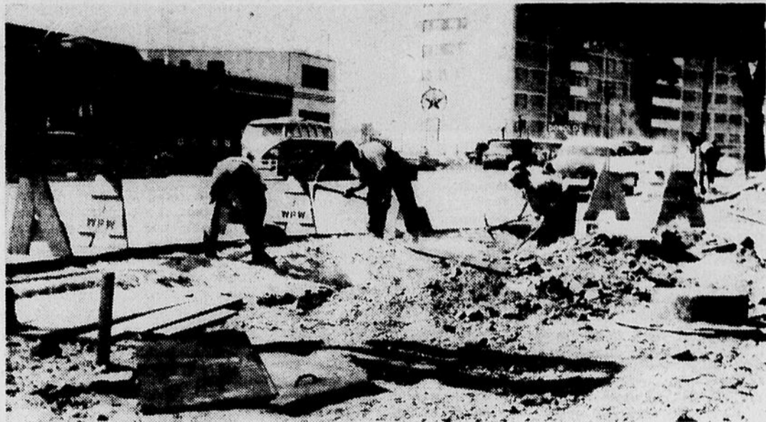
FINISHING TOUCHES: Contractors are busy clearing up the last bit of work on Victoria between the Boulevard and Sunnyside in preparation for the
