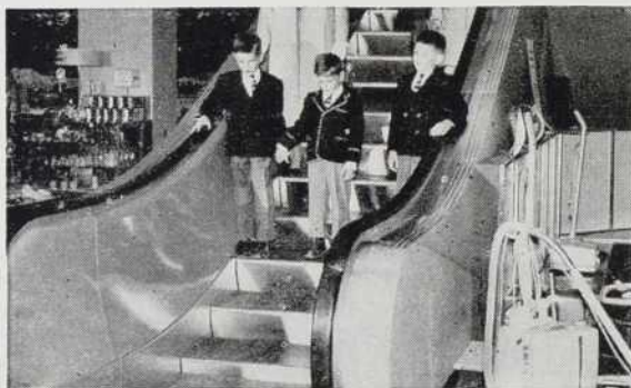
Simpson's-Sears Ltd. — Ent. Gén.: Commonwealth Construction Co. Ltd., Winnipeg. Arch.: Green, Blankstein, Russell and Associates, Winnipeg.
