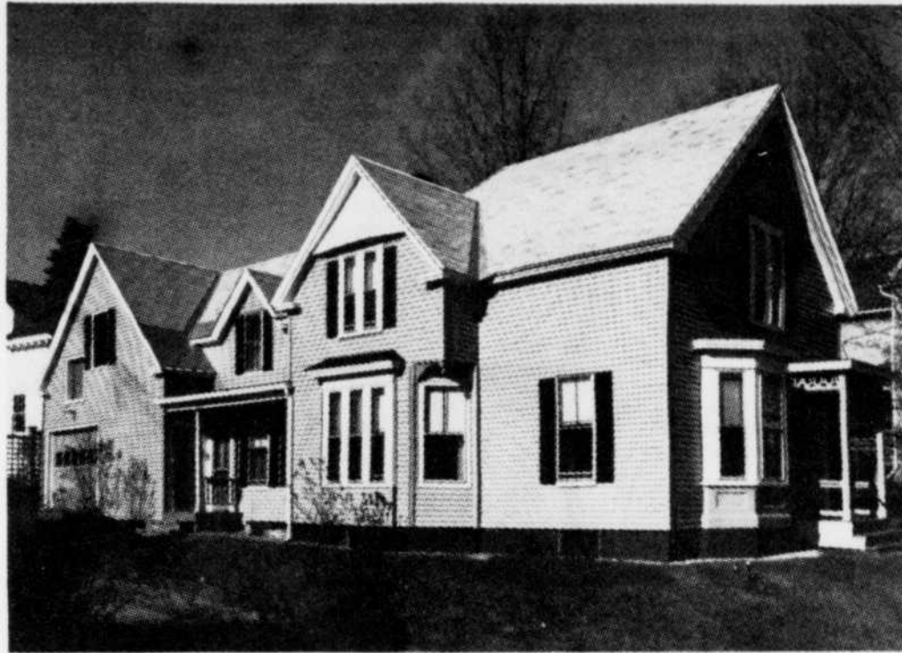
PRE-FINISHED SIDING does away with repainting costs and makes your old home look like new for years to come. This home built in the 1920's has been restored with tan aluminum siding. The old wooden window casings were covered with custom-formed sections of white aluminum to provide low maintenance while keeping the original style of the home. Other trim details (such as soffit, fascia, gutters and downspouts) are also white. Black aluminum shutters provide the final accent.
