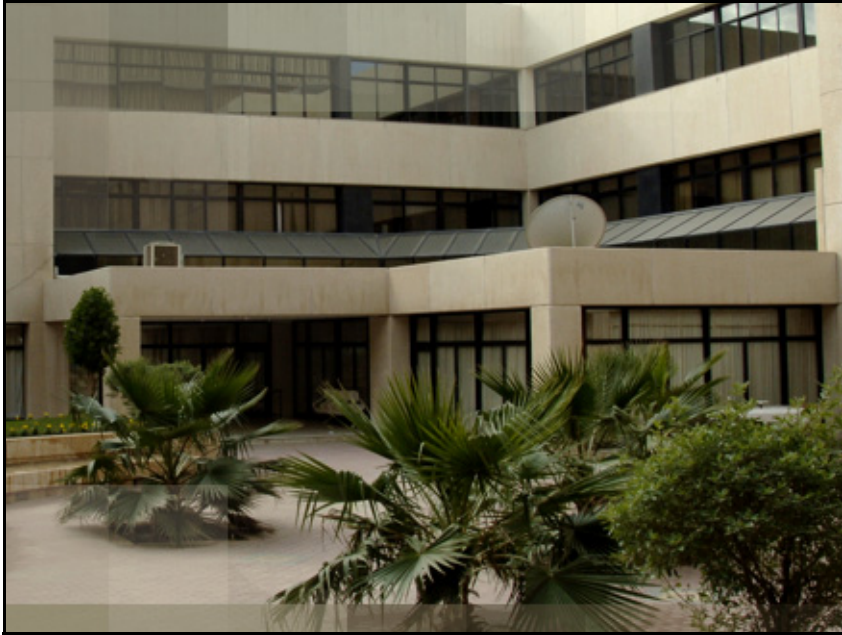
Figure 2.7: Department of Chemical Engineering.
