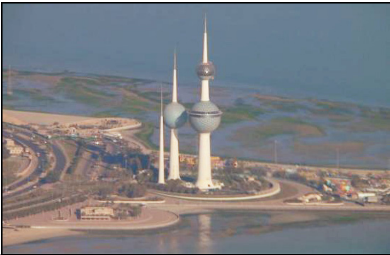
Figure 2.4: Observation towers in Kuwait City.
