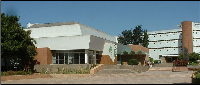
Figure 4.56: View of the Mohammadia School of Engineering.
