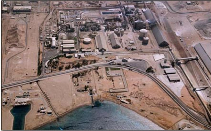
Figure 1.63: Fertilizer production plant.
