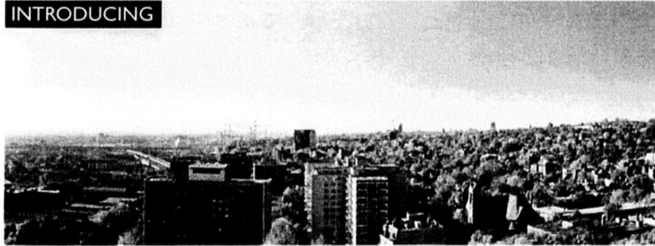
WESTMOUNT SQUARE | MLS 8642923 $3,500,000 Exceptional opportunity to own a unique unit of approx 5,000 sq. ft. on the 18th floor, all on one level in renown landmark property - Westmount Square. The spectacular east, south and western exposure offers an incredible 270 degree panoramic view, 4 parking spaces.
