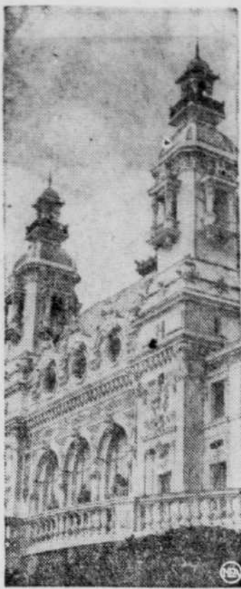
MONACO MECCA is the towering Monte Carlo Casino.
