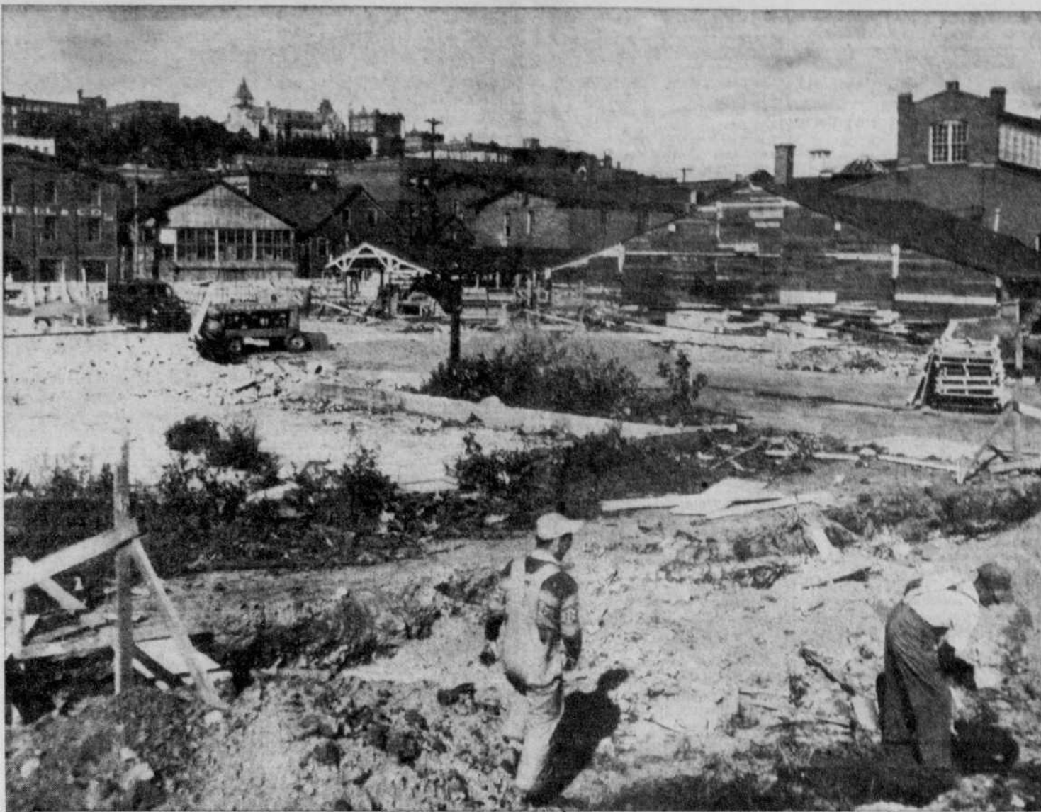
Market Construction — Work got under way last week on the new Lansdowne Market. After tearing down all obstacles, workmen are shown above preparing the way for the new foundation. (Record Photo by Gerry Lemay)
