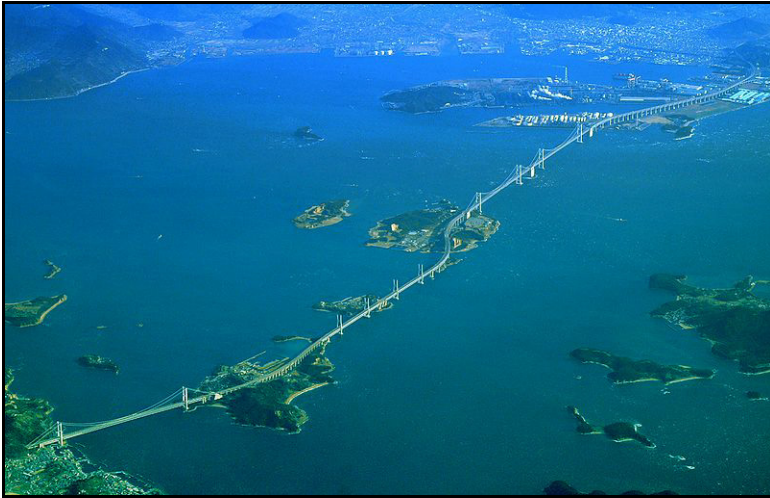
Figure 1.105: General view of the Great Seto-Ohashi Bridge.
