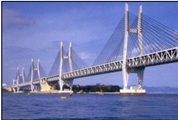
Figure 1.106: Another view of the Great Seto-Ohashi Bridge.
