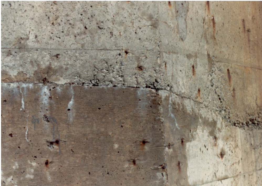
Photo 4.2-6 – Joint froid
