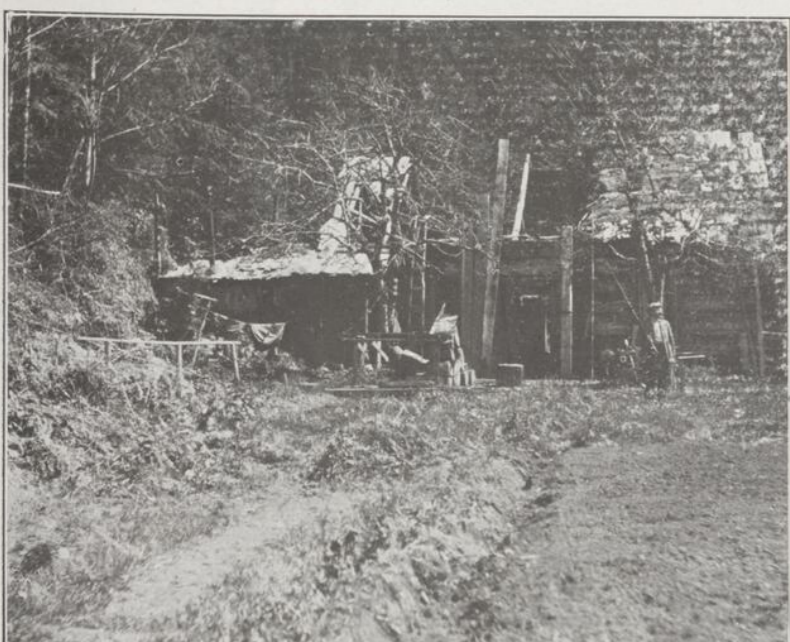
A CRUMBLING GUBERNATORIAL MANSION—Headquarters at Leechtown, B.C., of Governor Kennedy, now partially utilized by a Chinese miner.
