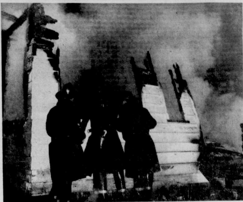
FLASH FIRE — A flash fire on the Beau Site road at Deauville Saturday night completely destroyed this bungalow, the residence of Emilien Dubreuil. Firemen from Sherbrooke fought the blaze. (Record photo by Gerry Lemay).
