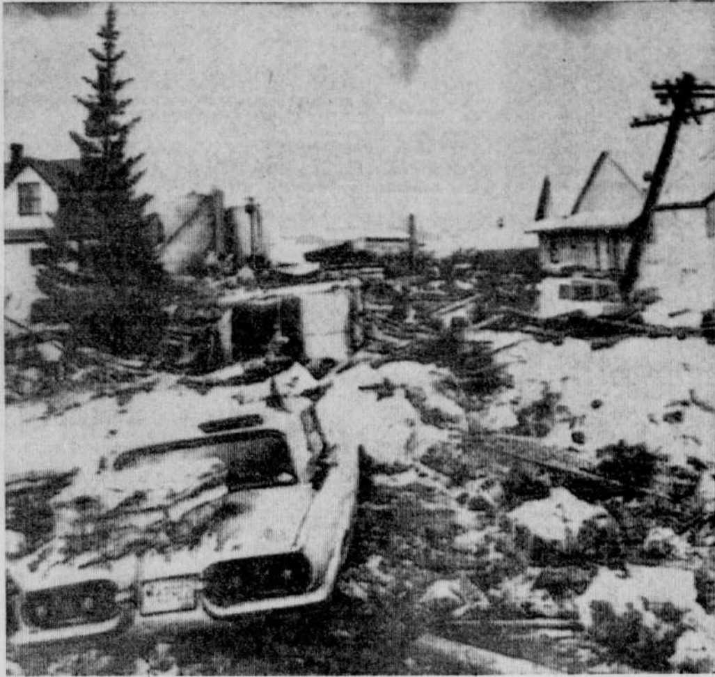
WRECKAGE AT VALDEZ — This was the ruin at Valdez where the earthquake struck with deadly force. Cars were buried and overturned by huge slab of ice pushed ashore by tidal wave which followed quake. (AP Wirephoto)
