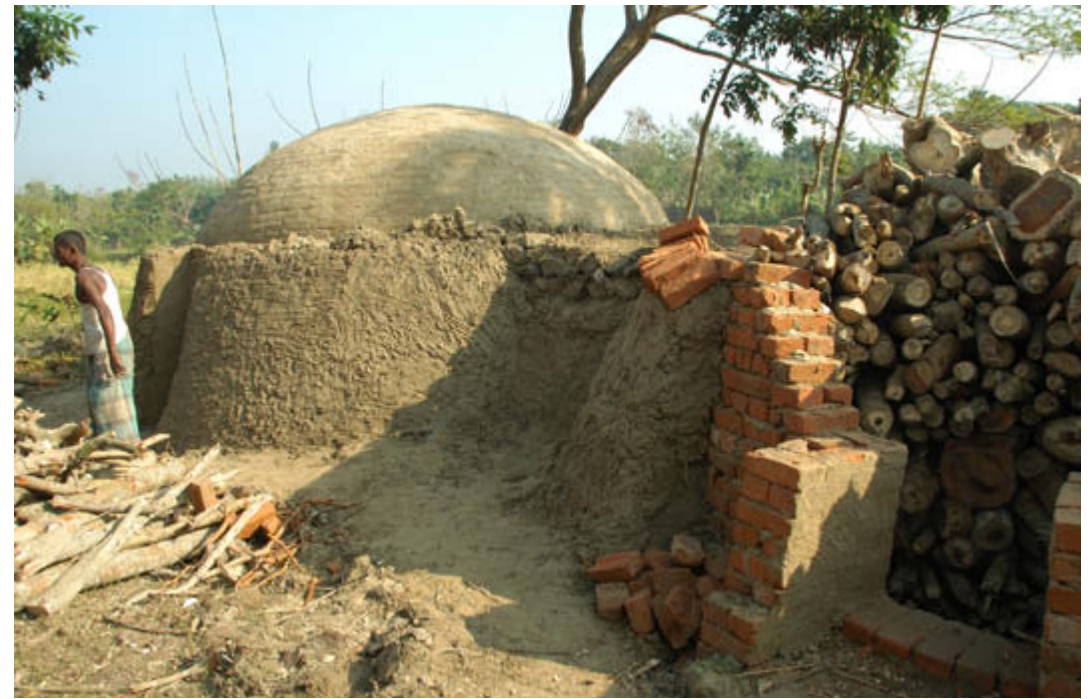
An artisanal brick-maker built this dome (a kiln) without formwork or cintering.
