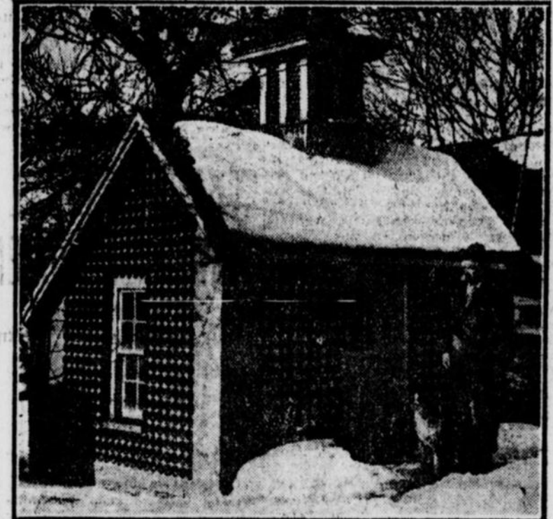
This house at Portsmouth, N.H., is entirely made of champagne bottles, there being 2,138 of them in all. The bottles were laid on their side with the bottoms out and cement filled in around them
