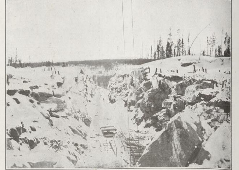
RAILWAY CONSTRUCTION IN CANADA—One of the large cuttings on the G.T.P. between Fort William and Winnipeg.
