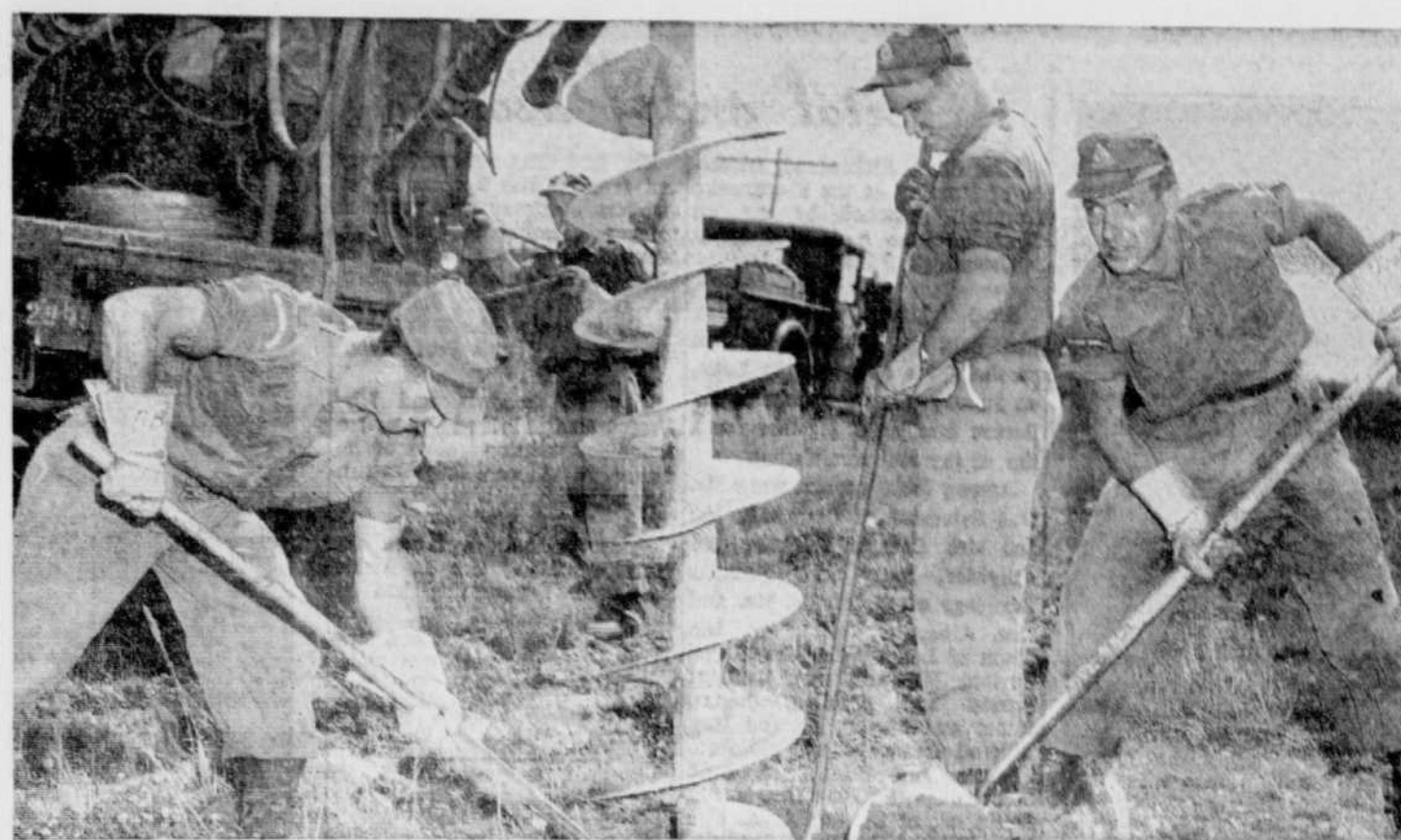
POLE PLANTERS — Signalmen of the Camp Gagetown Signal Troop, Royal Canadian Signals, sink a drill into the Camp Gagetown earth to erect a telephone pole for communications throughout the big training camp's 427 square miles. Left to right are Signalmen George Bailey, whose wife, Violet, lives at 374 Brock Street, Kingston, Ont., Signalman Gaston Courchesne, Sherbrooke, Que., and Signalman Roy McMullin, son of Mr. Malcolm McMullin, Reserve Mines, Cape Breton, N.S. (National Defence Photo)
