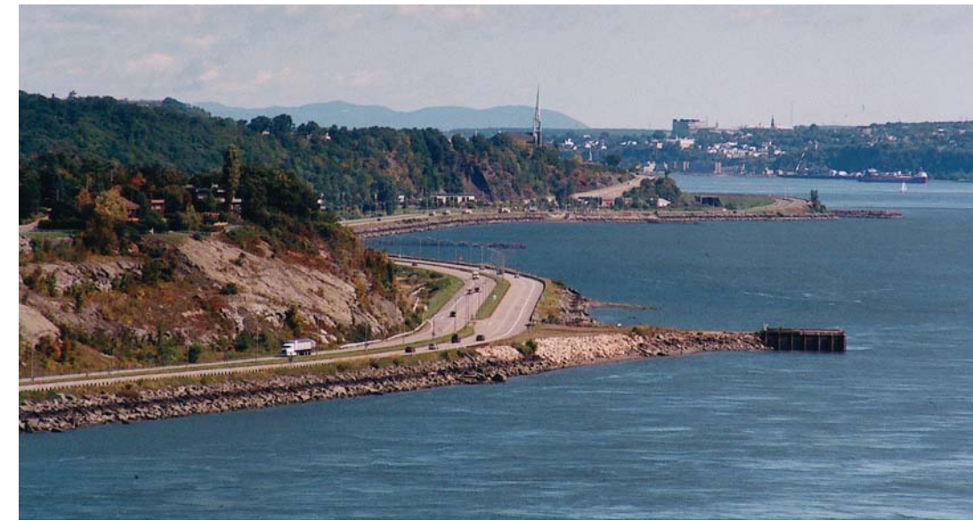
Interface between Champlain Boulevard, Foulon Road and the St. Lawrence.
