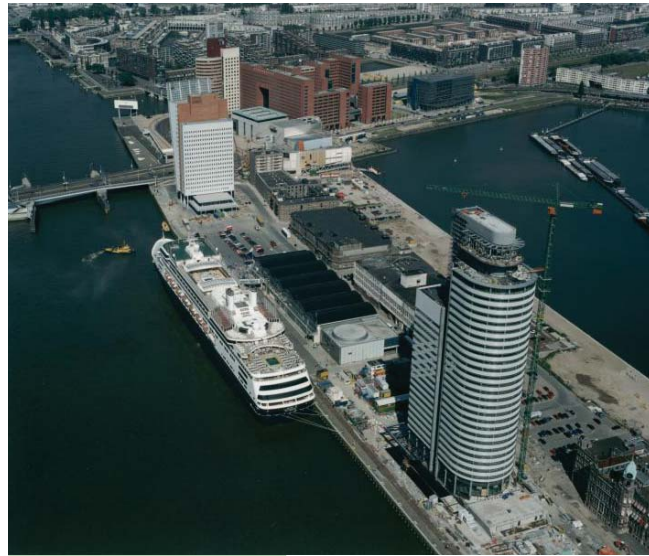
Aerial view of Wilhelmina Pier under construction.
