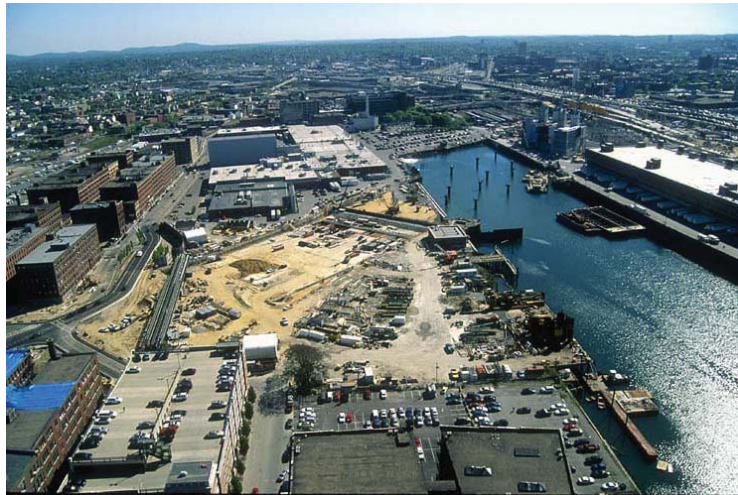
Aerial view of construction on the Fort Point Channel.
