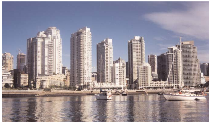
Concord Pacific Place, in the QuayWest area (along Marinaside Crescent).
