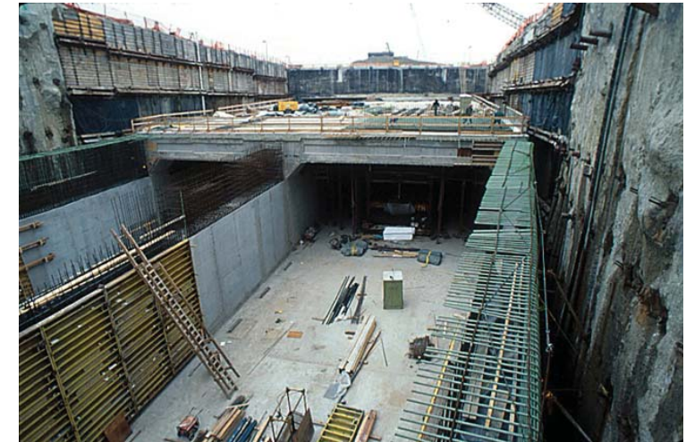
Construction of part of the tunnel in East Boston.
