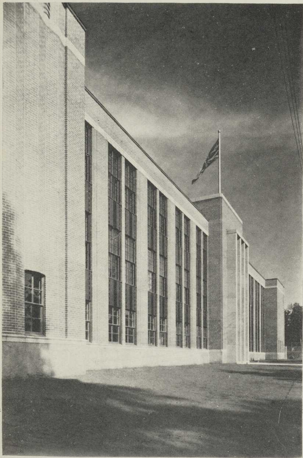
FRONT ELEVATION, QUEBEC HIGH SCHOOL, BELVEDERE ROAD.
