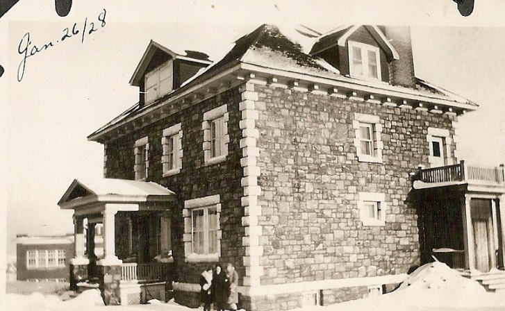
Rectory at North Bay
