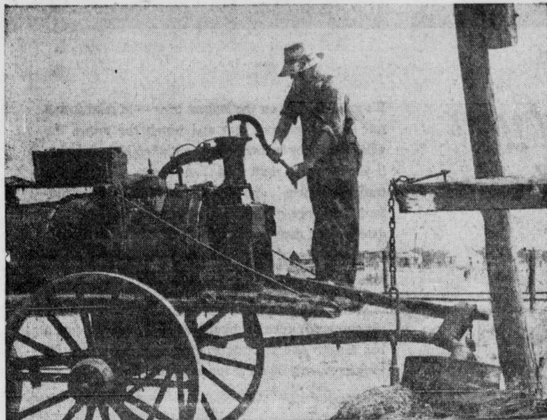
A small but steady income is garnered by local farmers who still work the wells on their land. Farmer above uses old-fashioned hand-pump to fill primitive wooden oil vat. Later, horse-drawn wagon will haul oil to pipe-line (said to be the first in Canada) feeding refinery at Sarnia.
