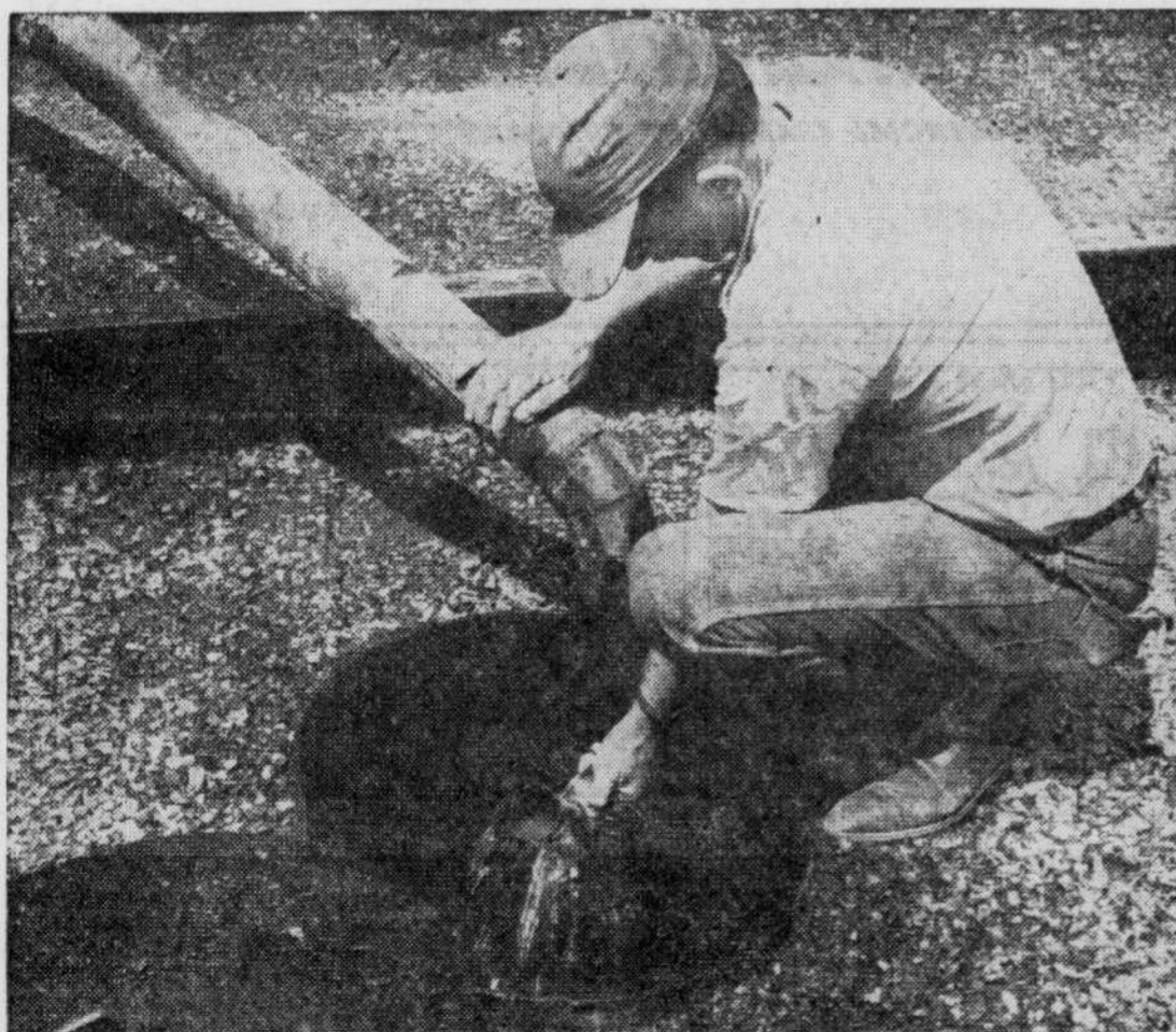
Today the busy refinery at Sarnia requires a mere 12 hours to process the annual output of the historic wells. Above, technician draws off sample from underground storage tank to test for specific gravity.
