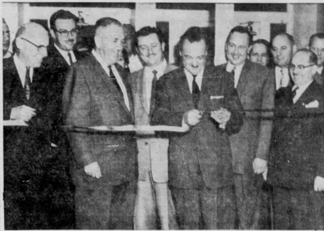
Bus Terminal Opens — Mayor Armand Nadeau cuts the ribbon officially opening the Laramie Bus Terminal on King st. west Saturday night. Looking on are Hon. J. S. Bourque, Alphonse Laramie, Jean-Paul Thibault and Alphonse Belanger. (Record Photo by Gerry Lemay)
