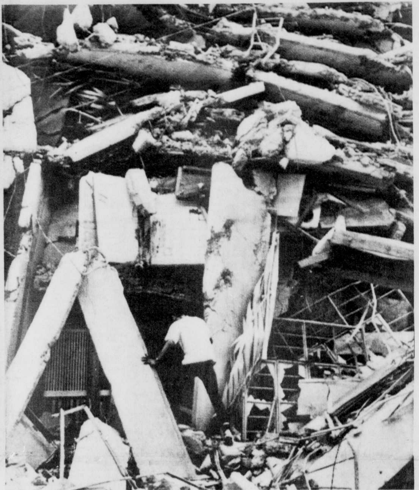
TRIES TO AID VICTIMS — A medical aide ventures under perilously hanging chunks of concrete, wood and other rubble to try and take medicine to trapped occupants in wreckage of apartment house in Manila, Philippines. The five storey building collapsed when a strong earthquake hit the area during early Friday morning when tenants were still asleep. (AP Wirephoto via cable from Manila)
