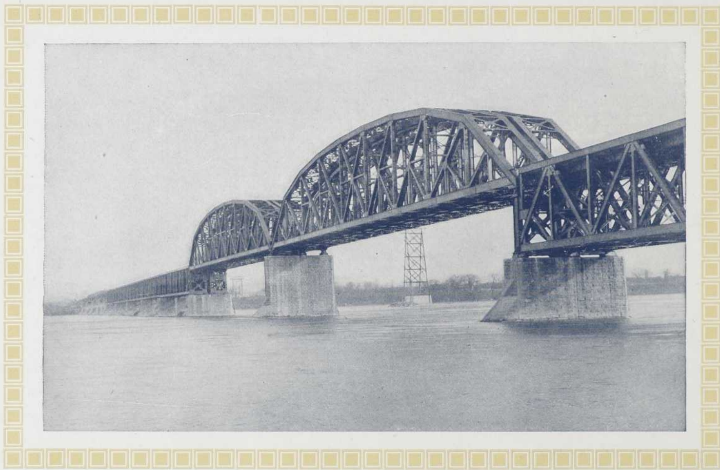
C. P. R. Bridge over St. Lawrence River—Near Montreal.
