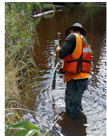
Installation of a piezometer in the riverbed
