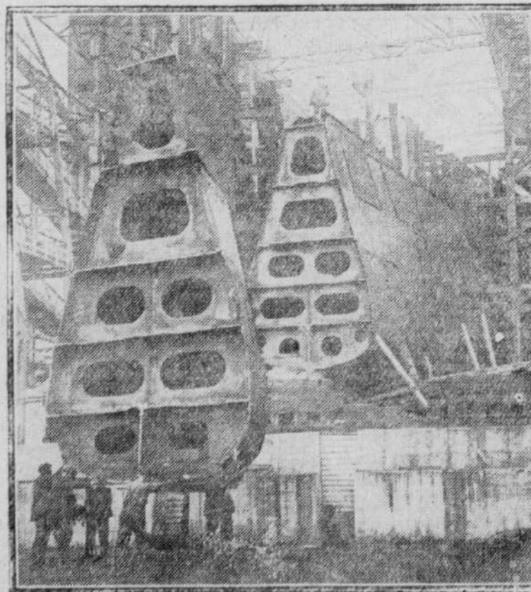
As though it were a piece of pie, the stem of the U.S.S. Indiana was sliced off the other day at the Brooklyn navy yards, where the battleship is being scrapped in accordance with the disarmament agreement
