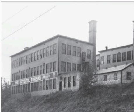
The first National Thread Company factory located on Laurier Avenue in Sherbrooke, in a building leased from the City of Sherbrooke. This factory location opened in 1941 and closed in 1952.
