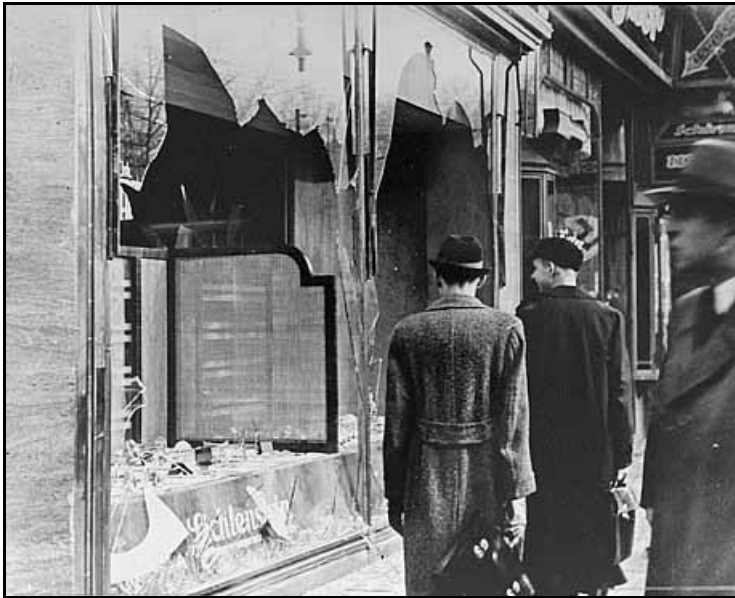
Figure 2.2: Glass windows smashed.
