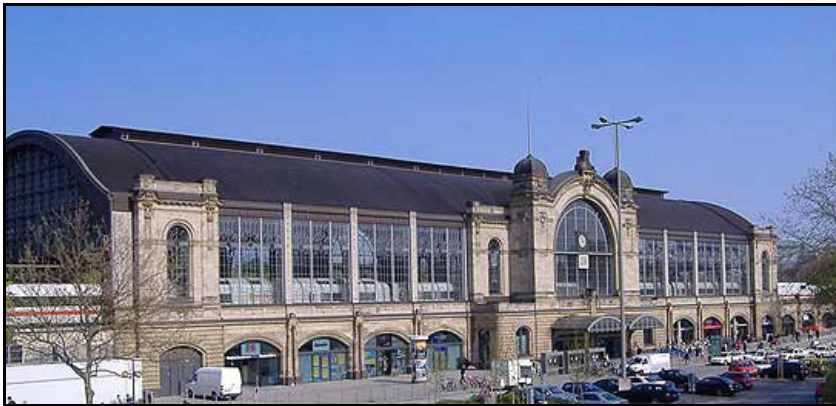
Figure 6.168: Dammtor Railway Station.
