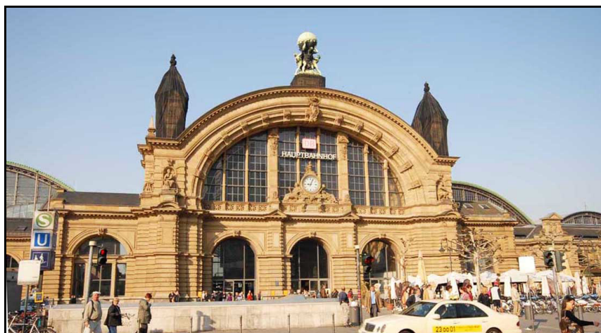
Figure 3.12: Frankfurt Railway Station, 1955.
