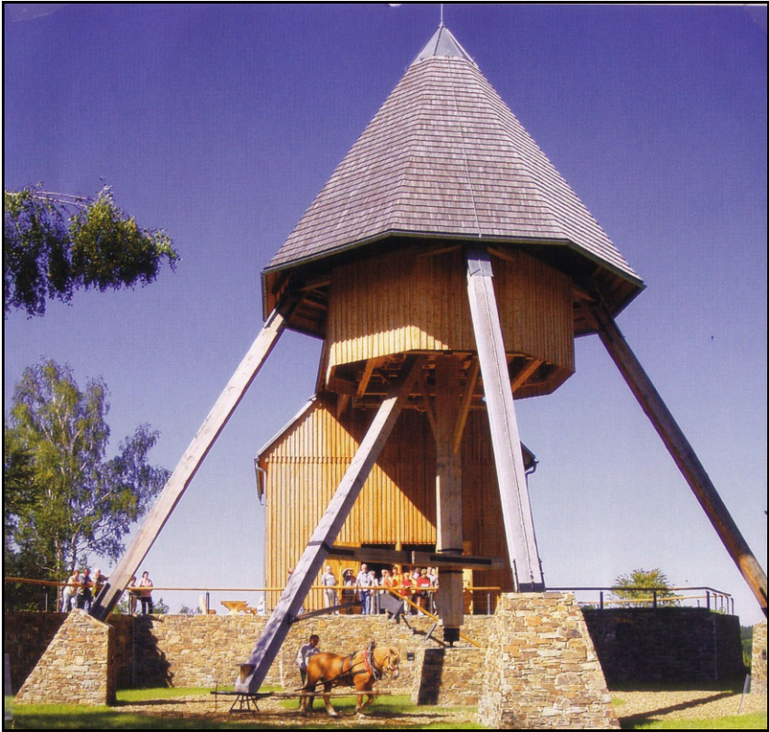
Figure 6.116: Horse capstan for ore transportation from mine at Marienberg.
