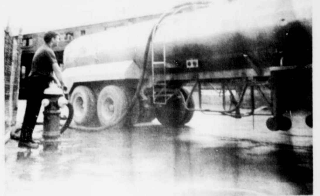
FOR AWHILE LONGER — Center on Stoke Road will continue to do so until the water pipeline linking Sherbrooke to the Medical center is fully installed and functioning.
