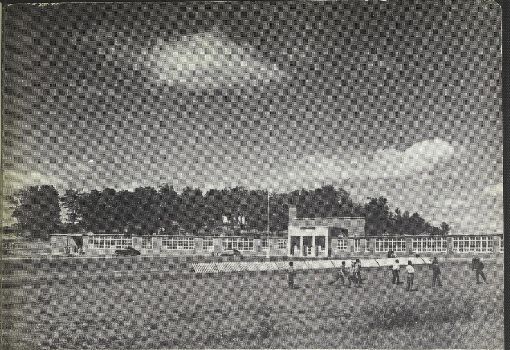
ASBESTOS-DANVILLE-SHIPTON HIGH SCHOOL
