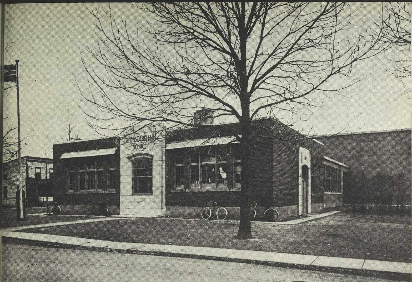
McMASTERVILLE INTERMEDIATE SCHOOL — EXTENSION AT REAR
