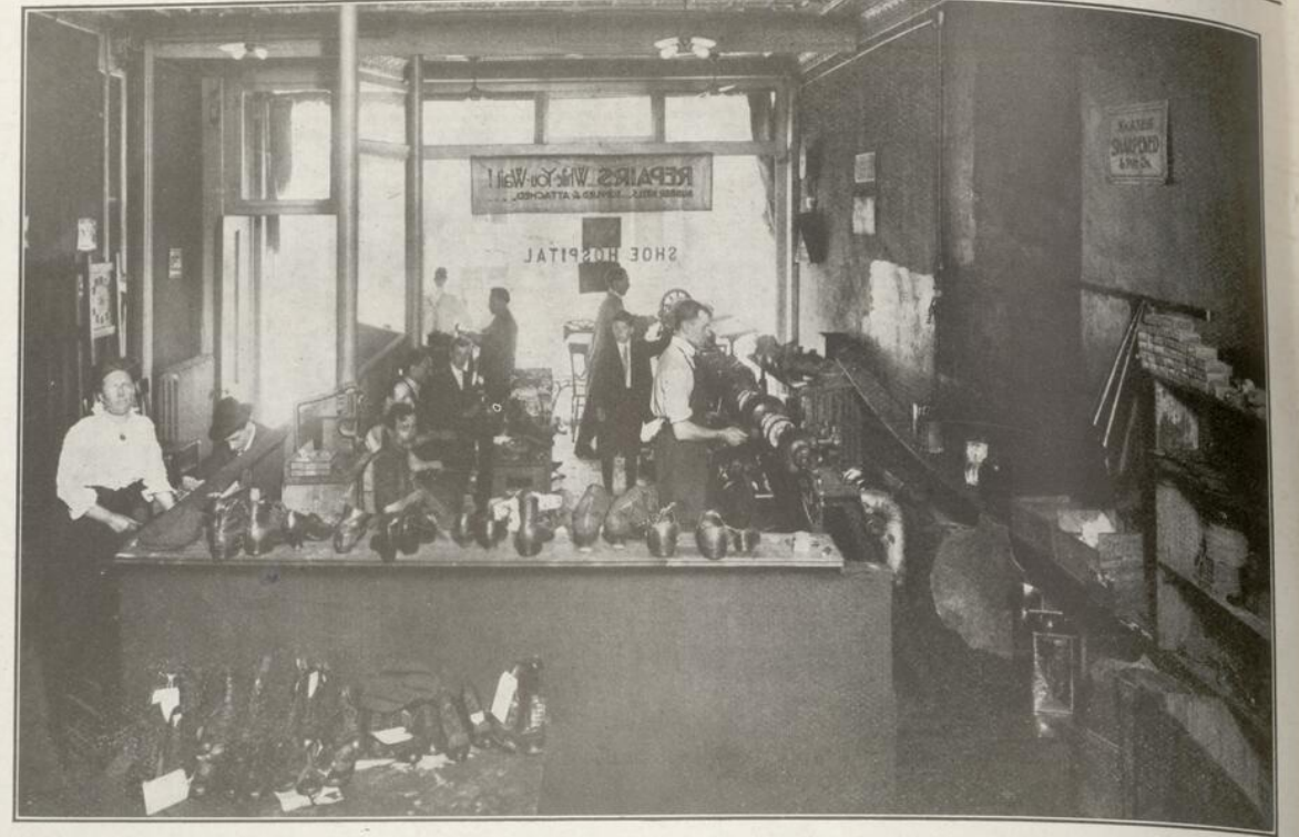
SUTHERLAND'S SHOE HOSPITAL, 389a BLEURY STREET.—Most people are loth to dispose of an old pair of boots or shoes, as it is always said that old boots are like old friends—and when such footwear is made to all appearances like new—few will dispense with footwear friends of long service and that explains the public patronage of this celebrated Boot and Shoe Hospital.
