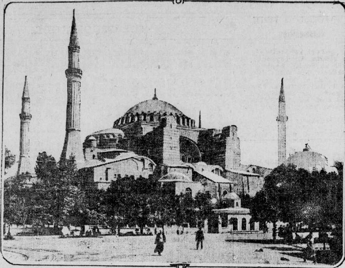
Greatest among Constantinople's 379 mosques is that of Agia Sofia, formerly the Church of Saint Sophia, which is 250 by 235 feet in size and was begun in the year 532. It was built in five years. Its shape is that of a cross. The dome in the centre rises to a height of 150 feet. In 1453 Mohammed II. changed the church into a mosque.
