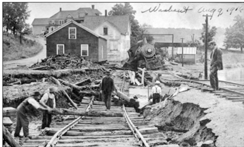
Railroad washout in Smith's Mills, August 9, 1916 (heritageogden.ca)
