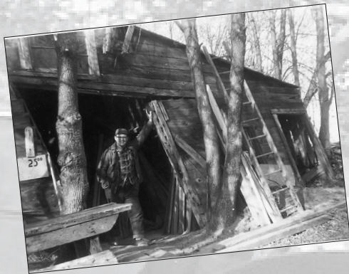
John outside their old sawmill building.
