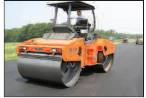
Figure 4 – Rouleau oscillant
