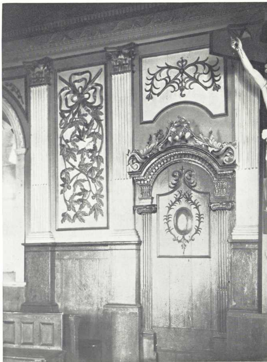
PART OF THE SOUTH WALL OF THE SANCTUARY
