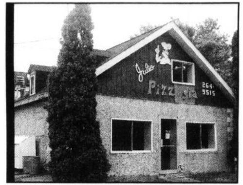
The building's last commercial incarnation was as a pizza restaurant.
