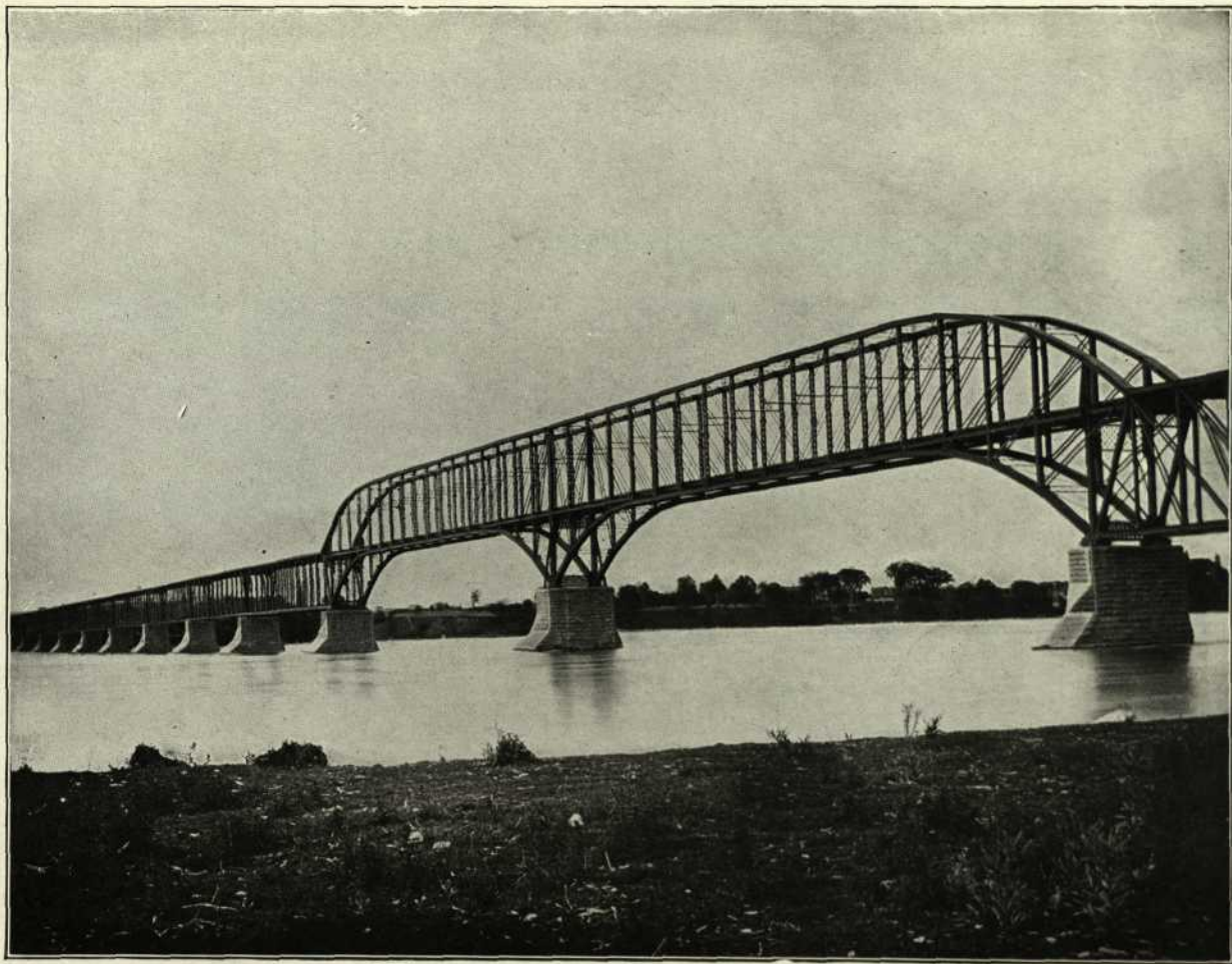
Canadian Pacific Railroad Bridge.
