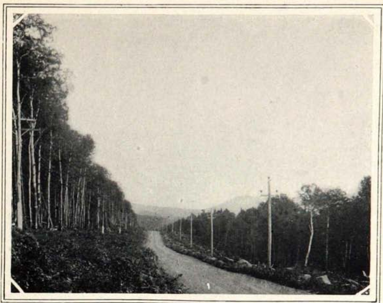
The Quebec-St. Siméon Highway, near St. Tite
