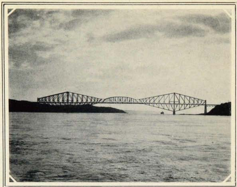
Quebec Bridge, longest single span bridge in the world
