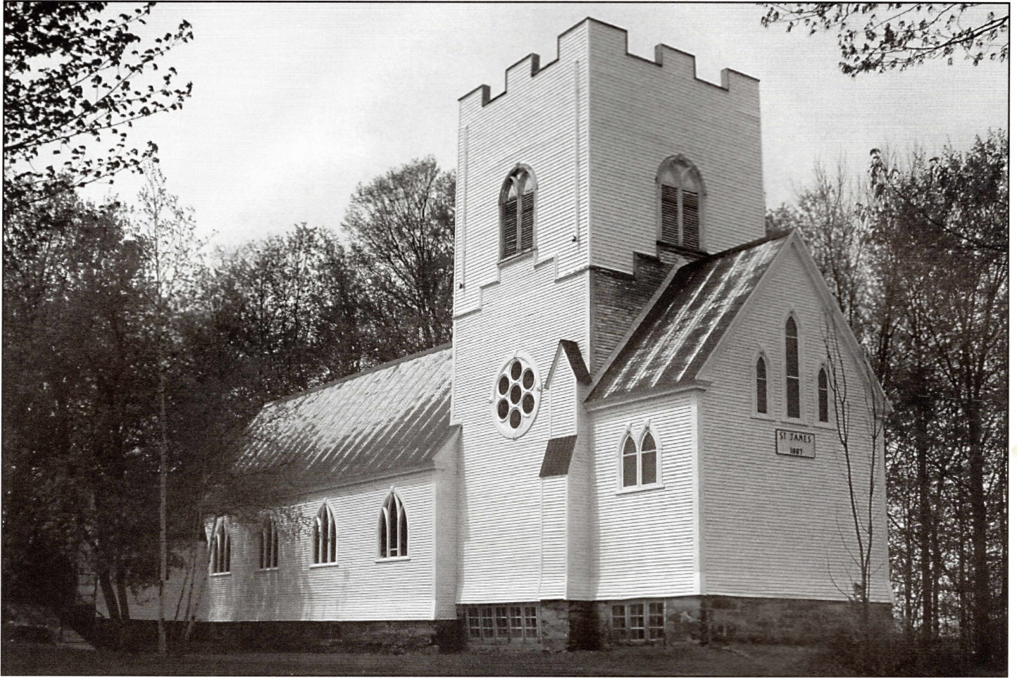
Compton's crumbling landmark, St. James the Less Anglican Church.
