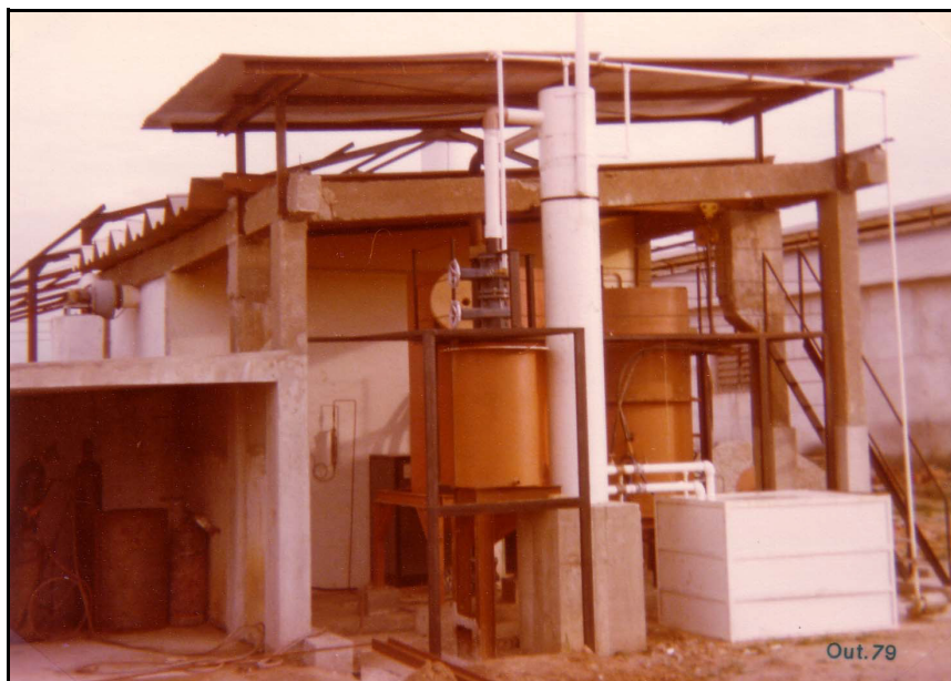
Figure 6.3: Pilot plant for the chlorination of pyrochlore at Lorena.
