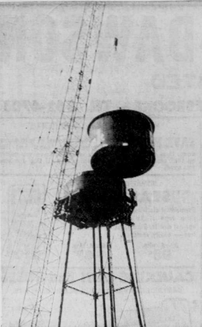
END OF 50,000 GALLONS — The water towers at Bruck Mills, Cowansville, have been landmarks for 63 years. According to company officials, the present tower was being dismantled because it had outlived its use as a means of fire prevention. The tank could hold 50,000 gallons of water and weighed 25 tons. Performing the dismantling operation is a 90 ton crane with a 150 foot boom. Cost of the operation was $5,000, said officials.
