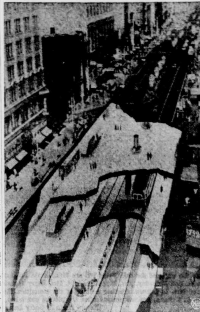
SUBWAY FOR SAN FRANCISCO — A subway planned for San Francisco is depicted in this combination photograph-drawing. The five-county Bay Area Rapid Transit District is developing the system which will be tied in with existing transit network. High-speed trains will use the subway's lower level while streetcars now operating on the surface will utilize central level. Upper level will be used for continuous pedestrian mezzanine where stations, escalators and entrances to downtown shops will be located. Similar subways are planned for nearby Oakland and Berkeley.
