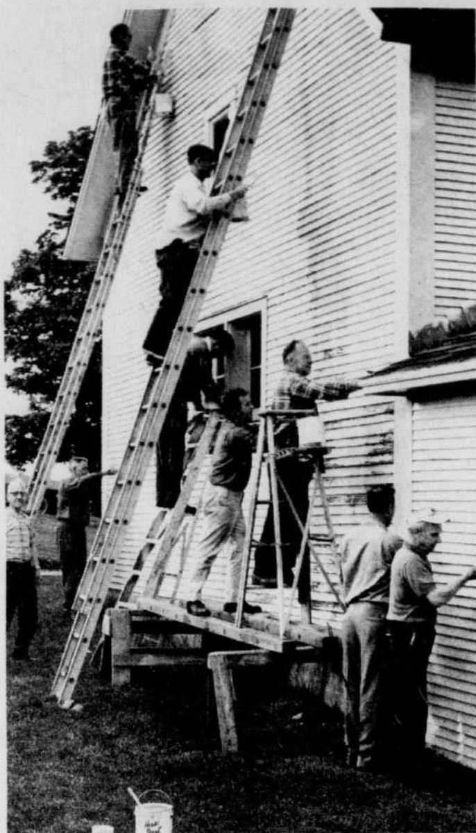
PAINTING BEE — The men of St. Paul's United Church in Waterloo organized an old fashioned work bee to spruce up the manse in time for the church's centennial in October. About 20 men worked on different nights to give the large house a fresh coat of cream colored paint. The job was started on June 10th and was finished on June 18th. (Record photo: Marcel Cote)
