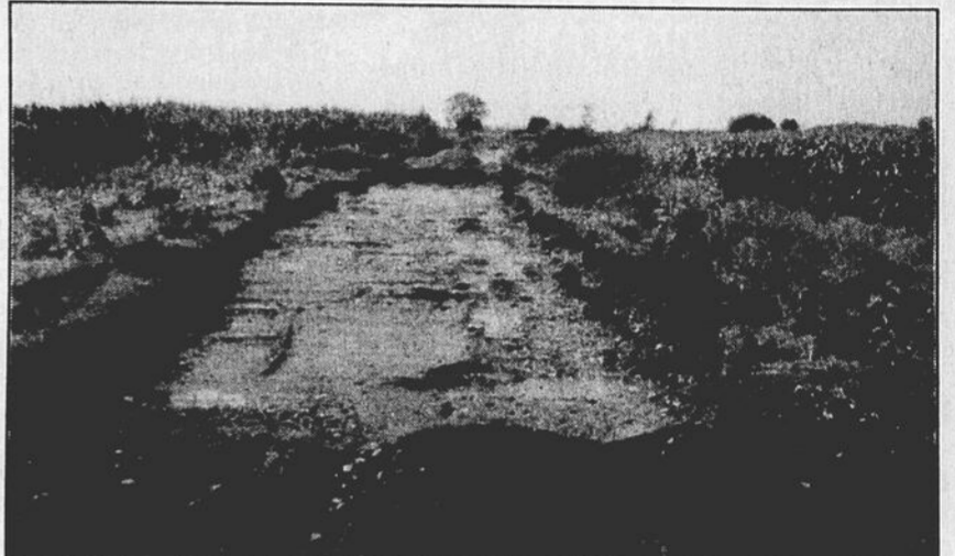
Part of the excavated portion of the rail line on the Michel Hébert farm in Trés-St-Sacrement, looking from the Tullochgorum Rd. toward Rte. 138.
