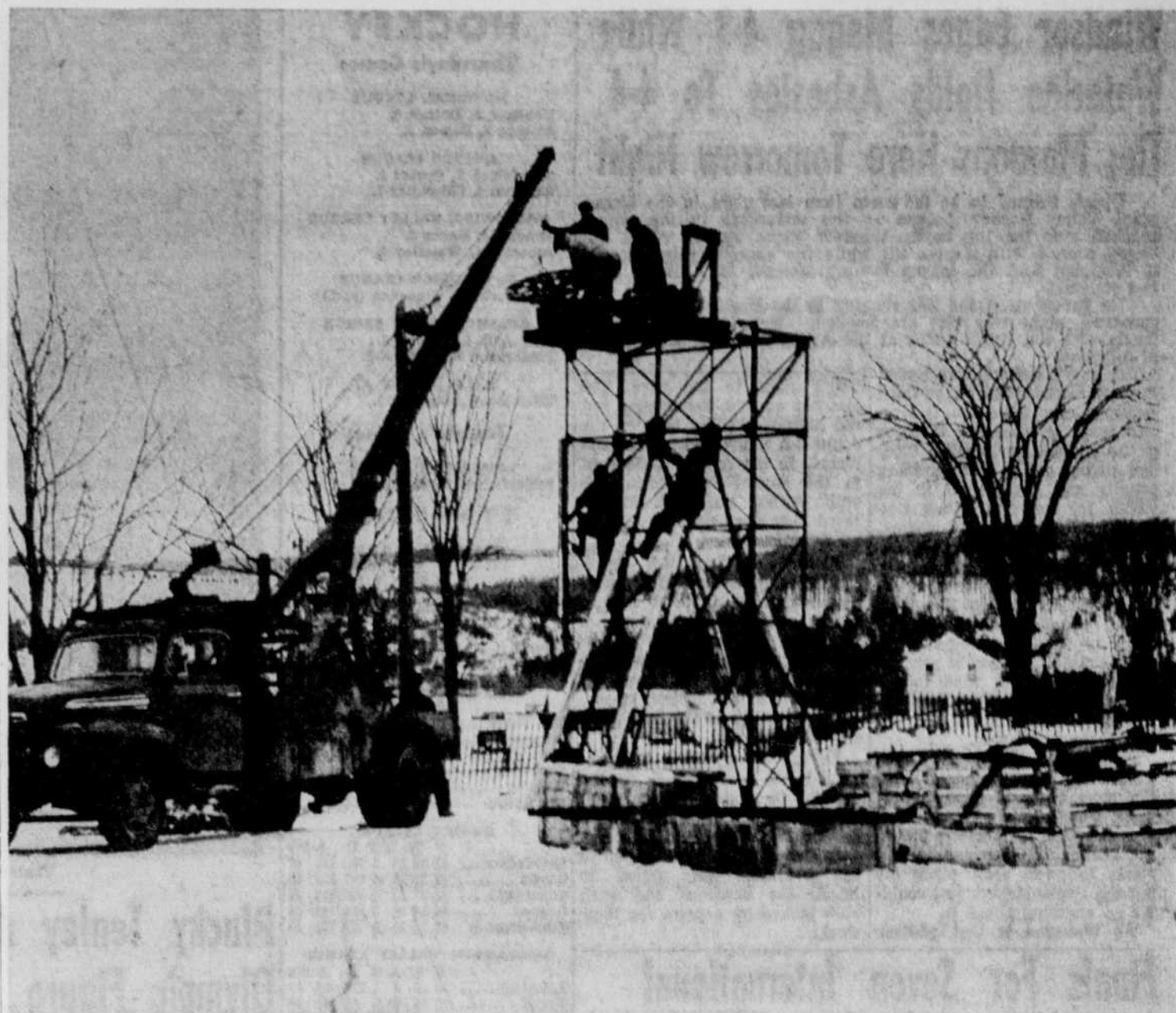
Workmen near completion on the erection of Hillcrest's new "Pomagalski" ski-lift which is to start running this weekend. The French-designed lift will have over a mile of rope and has a capacity of carrying 700 people an hour.
