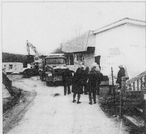
Camp Garagona under construction for purpose of expanding its respite services.
