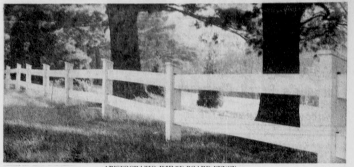
ARISTOCRATIC WHITE BOARD FENCE. (Record photos by Doug Gerrish)
