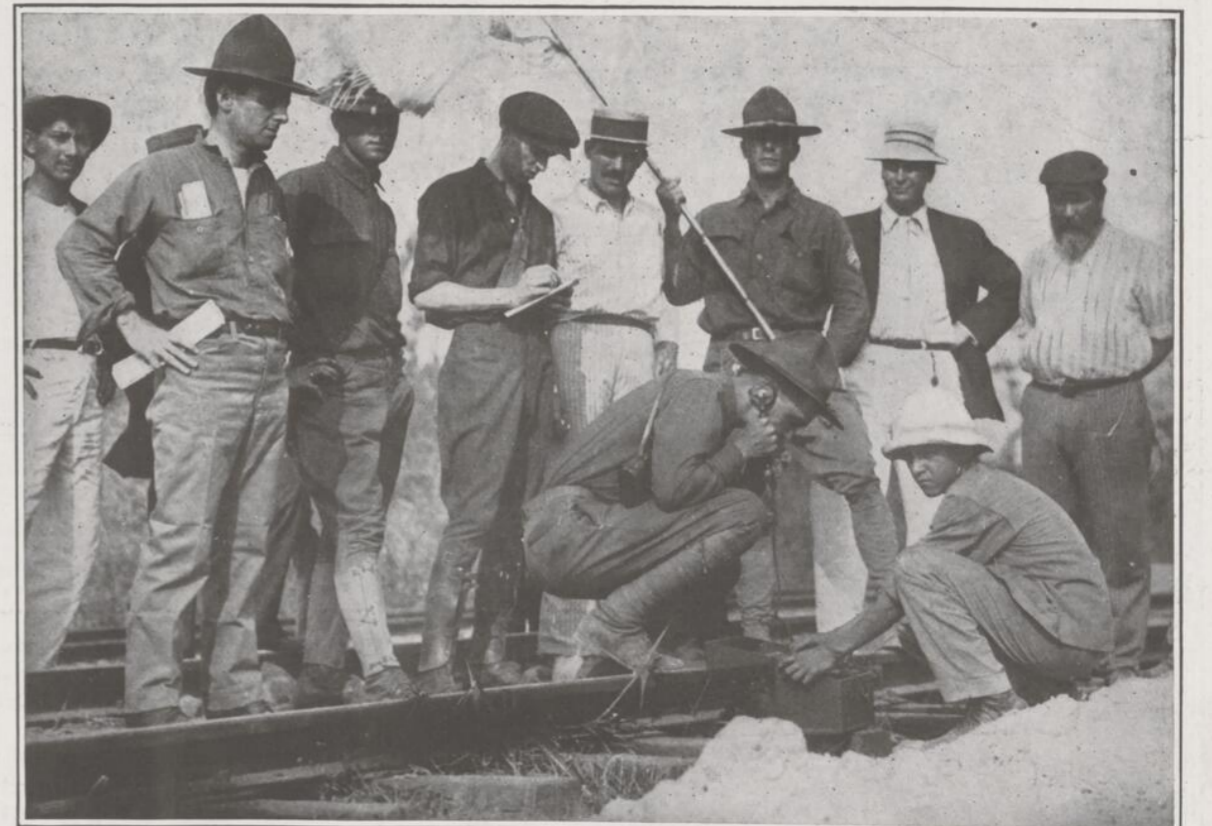
HOW AN ARMY MAKES TELEPHONE CONNECTIONS—Lieut. Richardson, of the United States Army, telephoning back to headquarters at Vera Cruz from the water works, (where he had held a conference with Major Sinancar of the Mexican forces), using the rails of the railway for conductors. (Copyright International News Service.)
