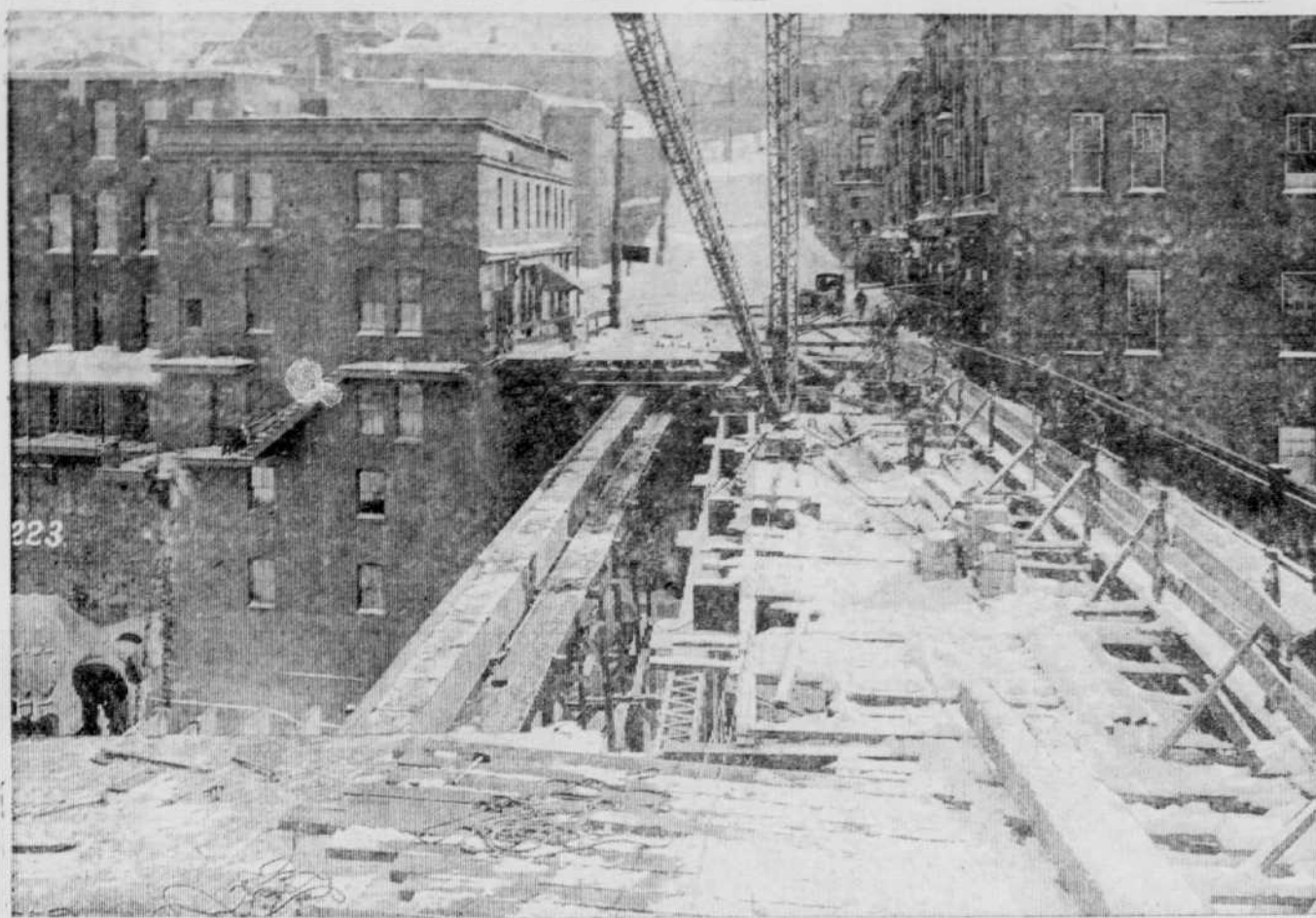
WORK PROGRESSES ON THE DUFFERIN STREET BRIDGE, MARCH 8, 1923.
